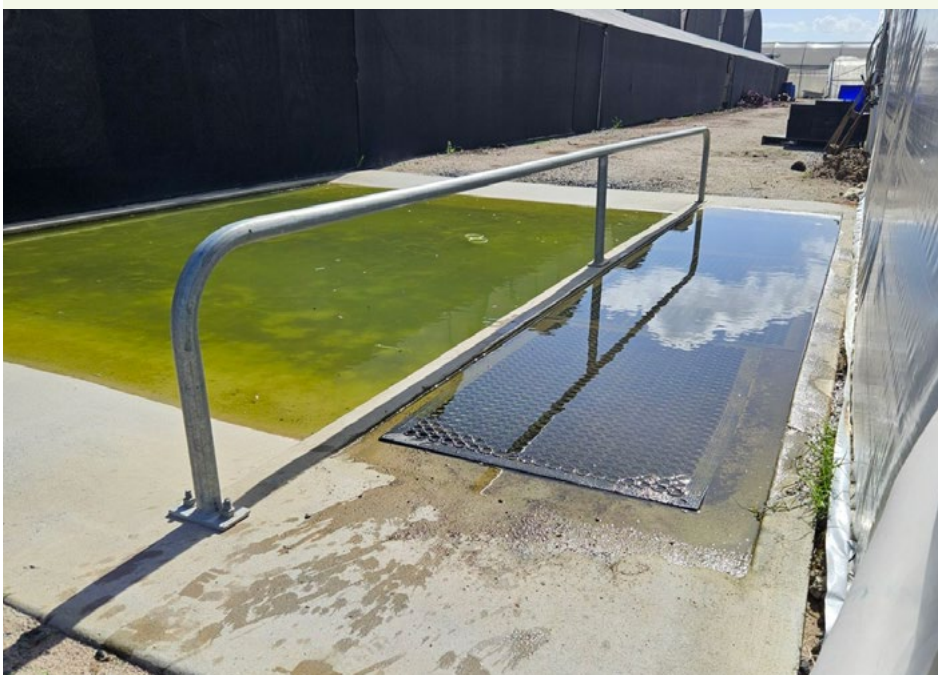
Dual foot bath and vehicle bath with safety rail.
